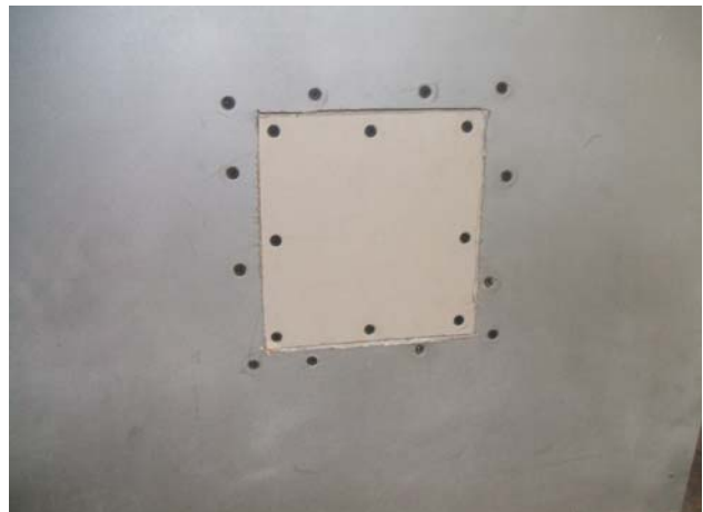
Figure 4. Apply Gypsum Board Patch
