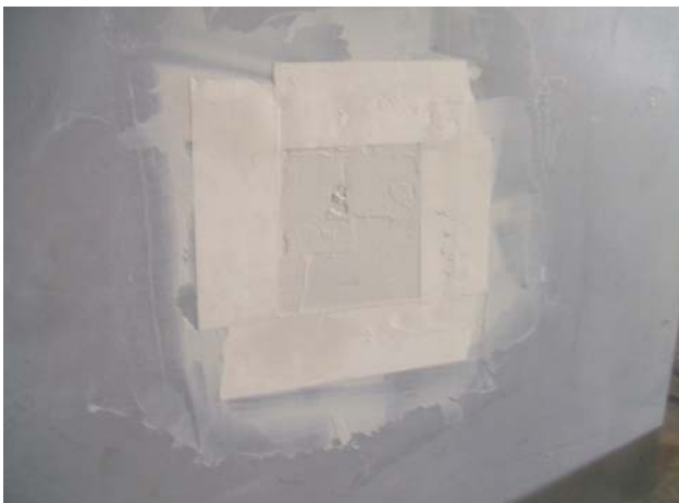
Figure 5. Tape and Finish Patched Area
