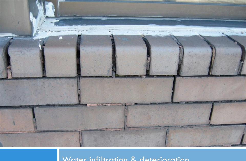
Water infiltration & deterioration
