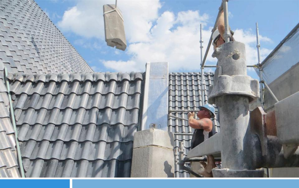
New through-wall metal flashing installed
