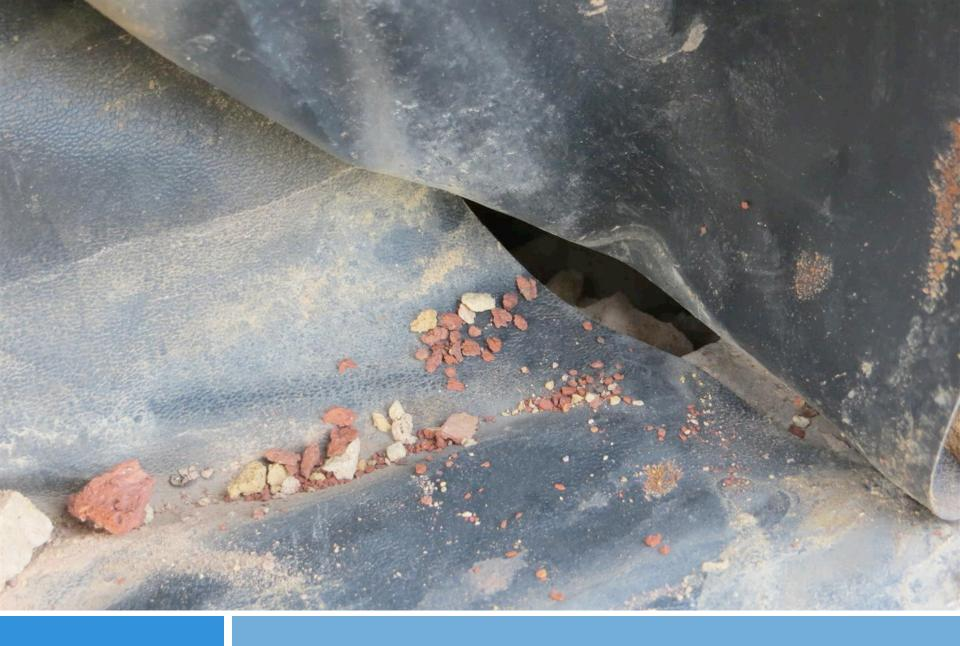
Plastic flashing was not sealed at lap joints
