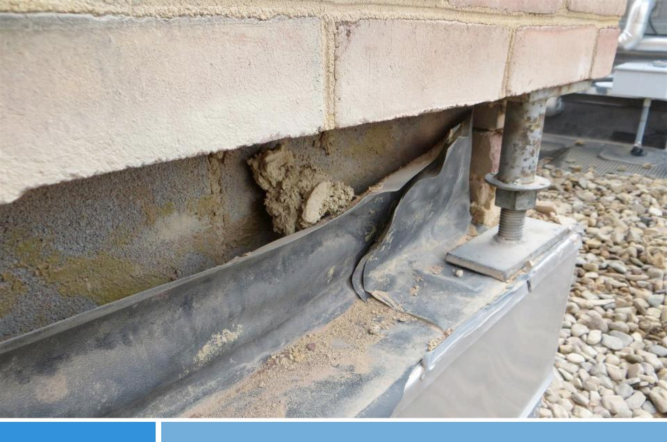
Flashing not properly terminated in the cavity
