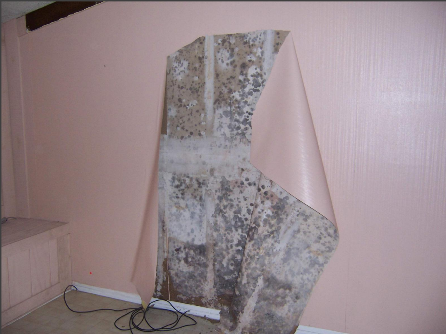
VINYL WALL COVERING AND MOLD
