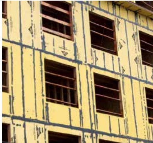
Sealed Gypsum Sheathing – Sealant Filler at Joints
