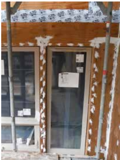
Sealed Plywood Sheathing – Sealant & Membrane at Joints
