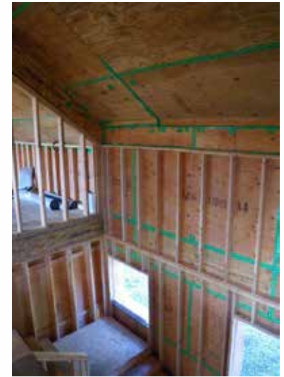
Plywood sheathing with taped joints (good tape)
