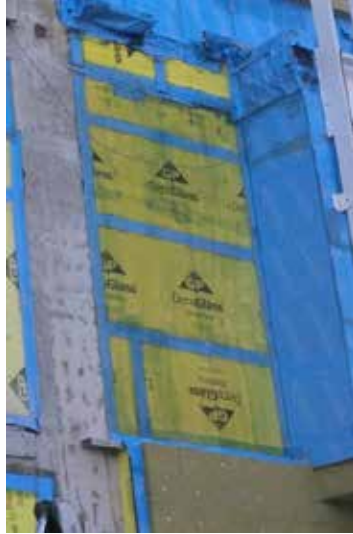
Sealed Sheathing – Membrane at Joints
