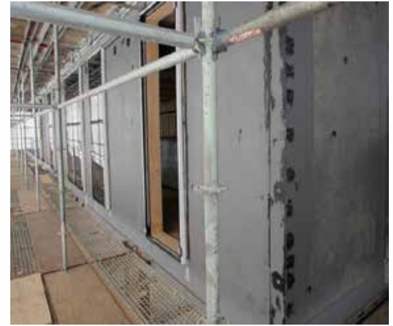
Liquid Applied – Silicone or hybrid sealants (STPE) and membrane
