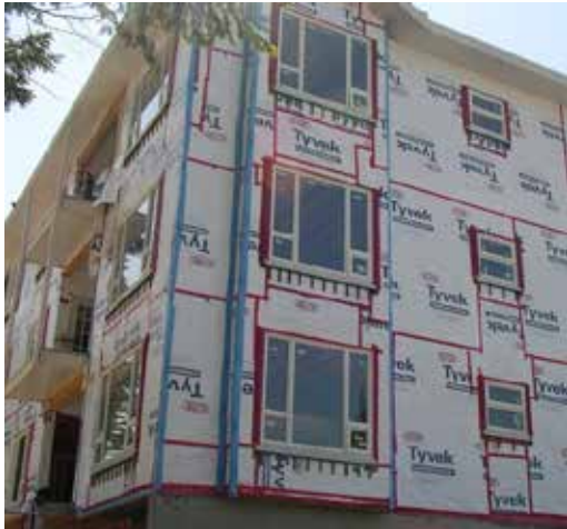
Loose Sheet Applied Membrane – Taped Joints & Strapping
